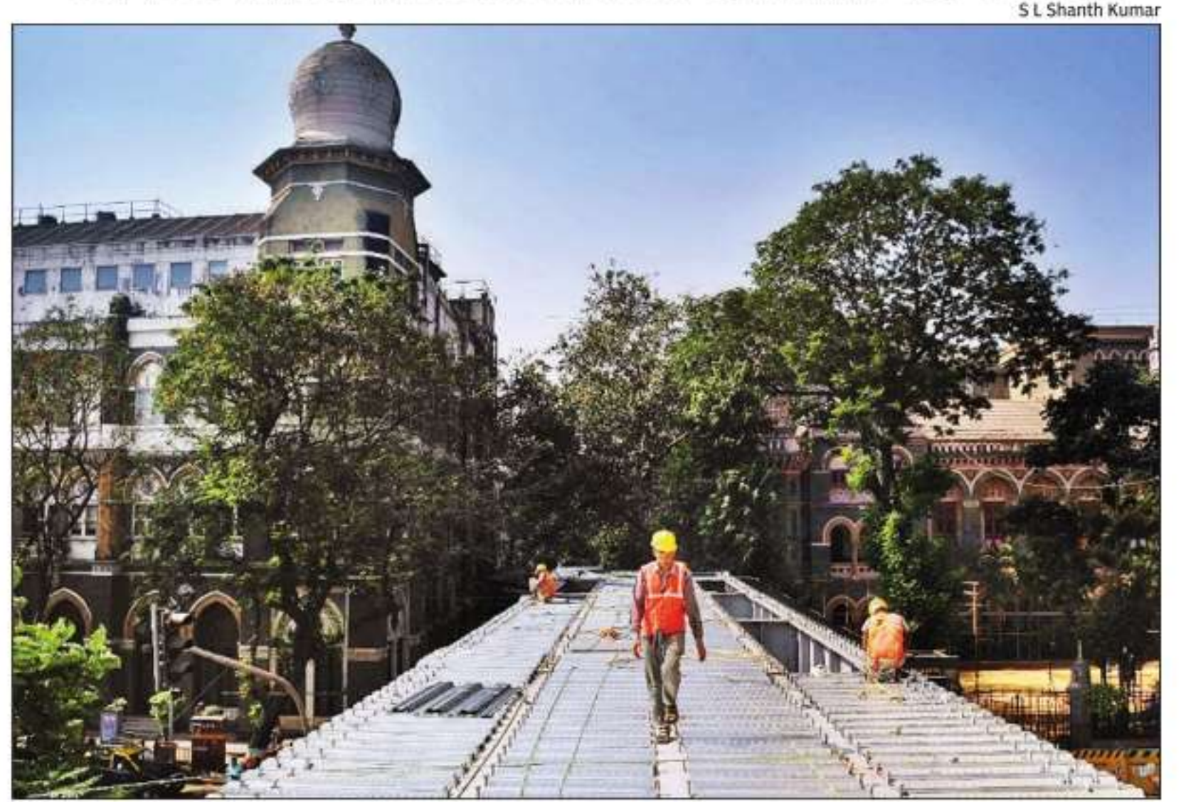
Three girders were launched earlier this month as part of Himalaya Bridge reconstruction. The bridge, which had collapsed in March 2019, killing seven people, is expected to reopen to pedestrians next month
