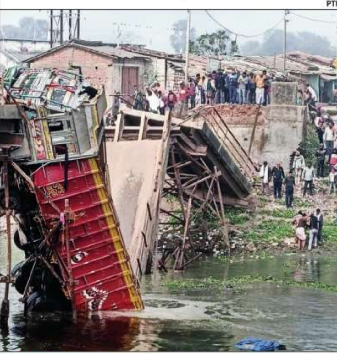
IN A ‘LORRY’ STATE: An iron bridge over Kamlia river in Bihar’s Darbhanga collapsed under the weight of a sand-laden truck on Monday. As the truck hung off the bridge, the driver and his helper were rescued. Activists said barriers had been placed to keep heavy vehicles off the structure built in 2004, but miscreants removed them
